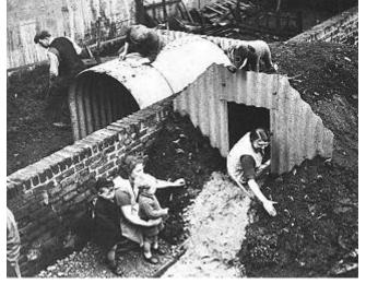
plates at either end. They measured 1.95m by 1.35m. The entrance was protected by a steal shield.
